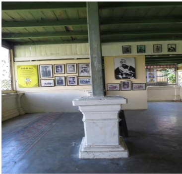
Fig. 6 Elevation of the timber column sitting on brick (left), the hybrid column footing when timber encounters masonry (right).
