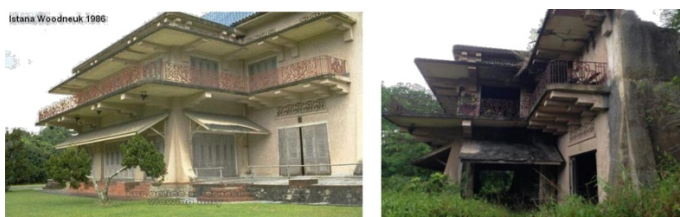
Fig. 10 The Woodneuk Palace: with extended ornamental balconies, lean to shading projections and corbelling forms and the elevated style with sinuous columns depict the Malay style, interpreted in a modern sense.
