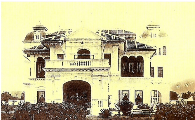
Fig. 1 The increasingly dominant Colonial expression onto Malay public buildings in Colonial Malaysia– as seen in one frontage of the Istana Hulu built-in 1896.
