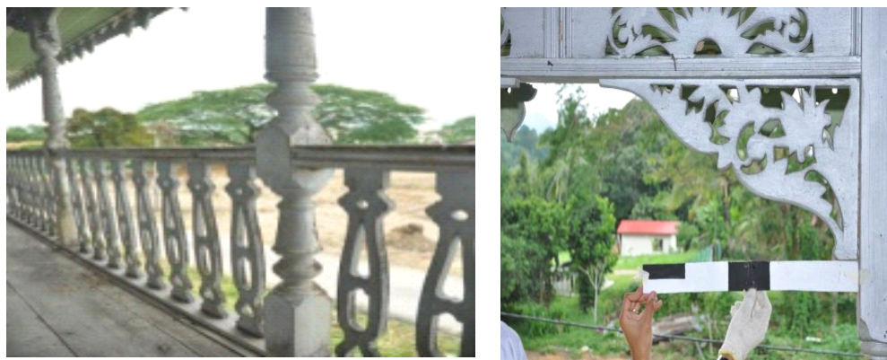
Fig. 13 Carved bracket and balustrades at the portico.
