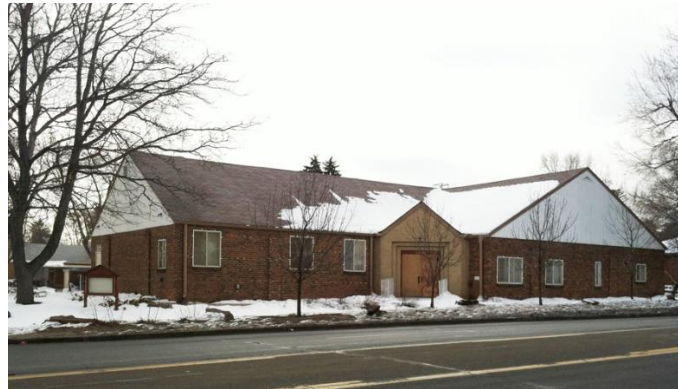
Fig. 3 Existing building before the renovation (Pel-Ona Architects & Urbanists)
